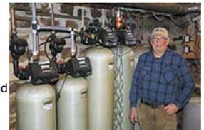
Greg Johnson uses eight water conditioner tanks to treat his farm's water. Johnson installed the conditioners after discovering a high level of iron, manganese and low pH were affecting his herd's health and production four years ago.
